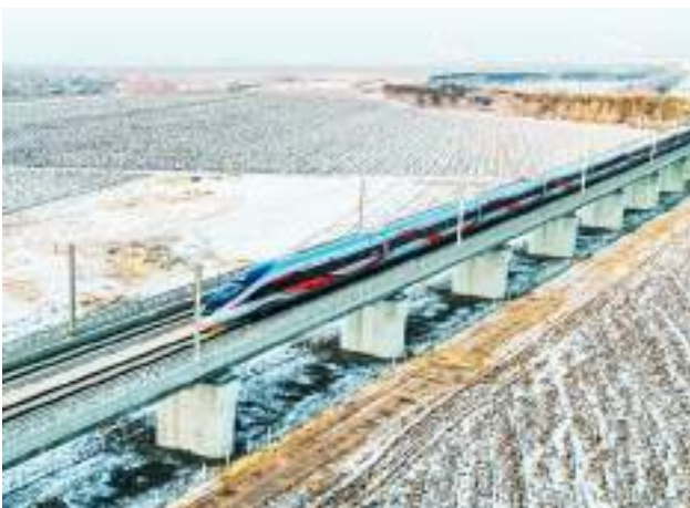
A4 Harbin-Dalian HSR: With a total length of 921 km and a design speed of 350 km/h, the Harbin-Dalian HSR opened to traffic in December 2012. It was the world's first operating HSR running in a very cold area with seasonally frozen soil.
