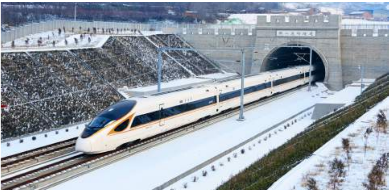
B6 New Badaling Tunnel (Badaling Great Wall Station): With a total length of 12.01 km, a maximum burial depth of 102 m and a maximum span of 32.7 m, this is the bored railway tunnel with the largest single arch span in China. It passes under the Badaling Great Wall twice and is located just 4 m away from the above-ground Qinglongqiao Station of the former Beijing-Zhangjiakou Railway, making the ancient majestic Great Wall blend in with the modern intelligent HSR.
