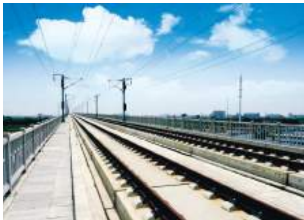
CRTS III slab ballastless track
