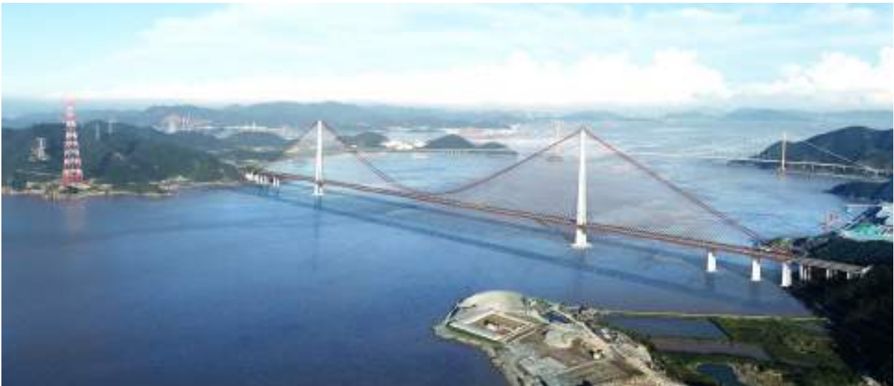
B5 Xihoumen Road-rail Bridge: Extending 3.1 km in length, this bridge features a main span of 1,488 m and employs a combined cable-stayed and suspension structure. Construction commenced in October 2022. It will be a rail-road bridge with the longest span of its kind in the world.
