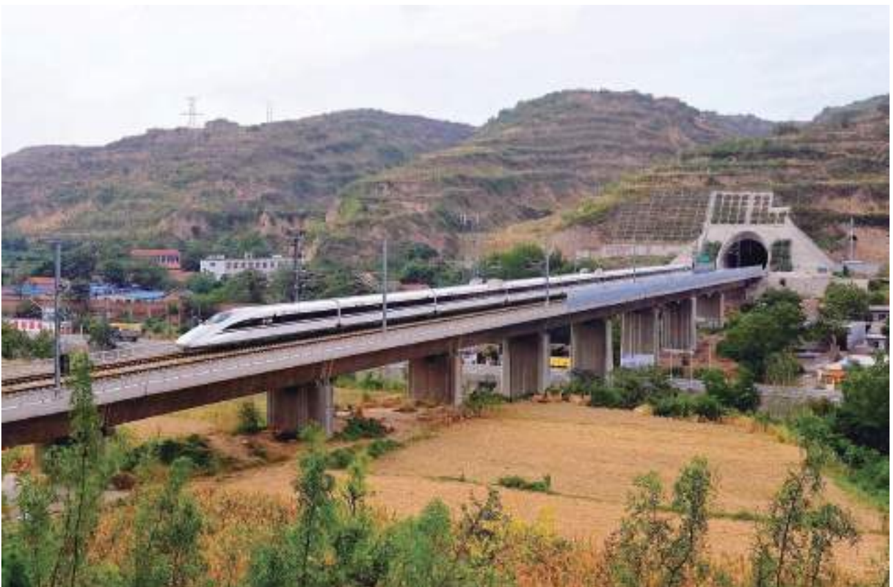
A2 Zhengzhou-Xi'an HSR: With a total length of 523 km and a design speed of 350 km/h, the Zhengzhou-Xi'an HSR was put into operation in February 2010. It was the world's first HSR built in a large collapsible loess area.
