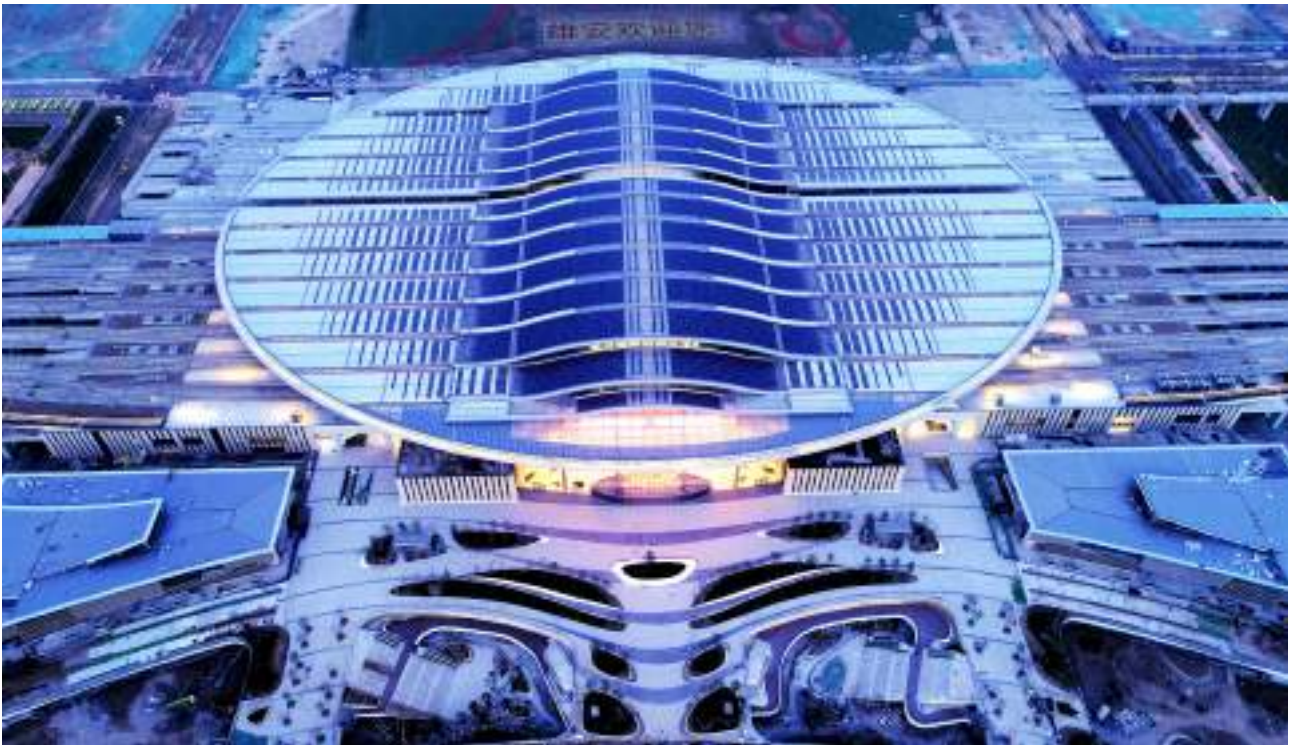
Xiongan Railway Station: With a total floor area of 475,200 m 2 , this railway station was designed under the concept of “station-bridge integration” and the passenger waiting area features a three-dimensional, two-storey layout. It is the first railway station in China to figure the extensive application of fair-faced concrete columns.
