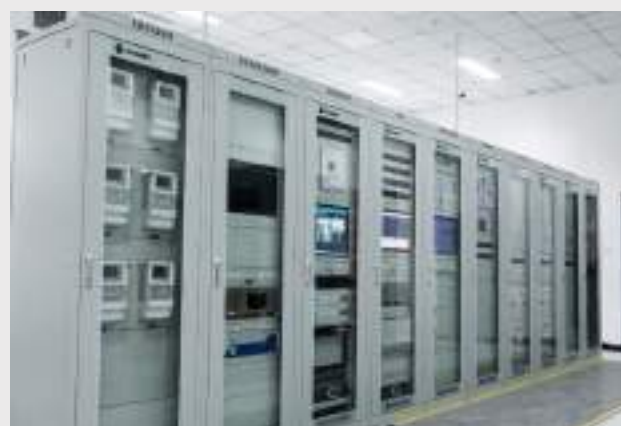
Intelligent wide-area monitoring and control protection system for traction substation
