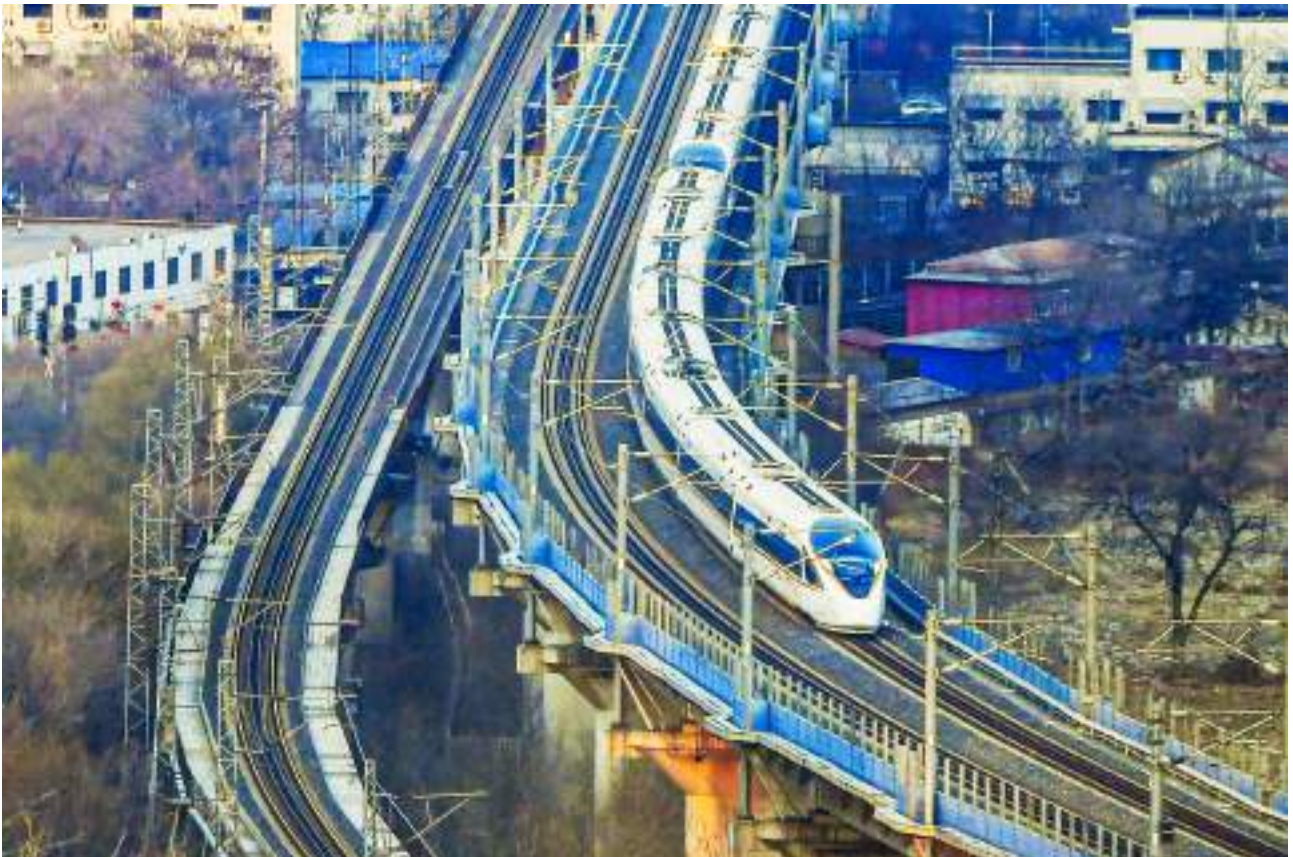
A1 Beijing-Tianjin Intercity Railway: In August 2008, the 120-km-long Beijing-Tianjin Intercity Railway was put into operation, making it an HSR reaching a design speed of 350 km/h for the first time in China.
