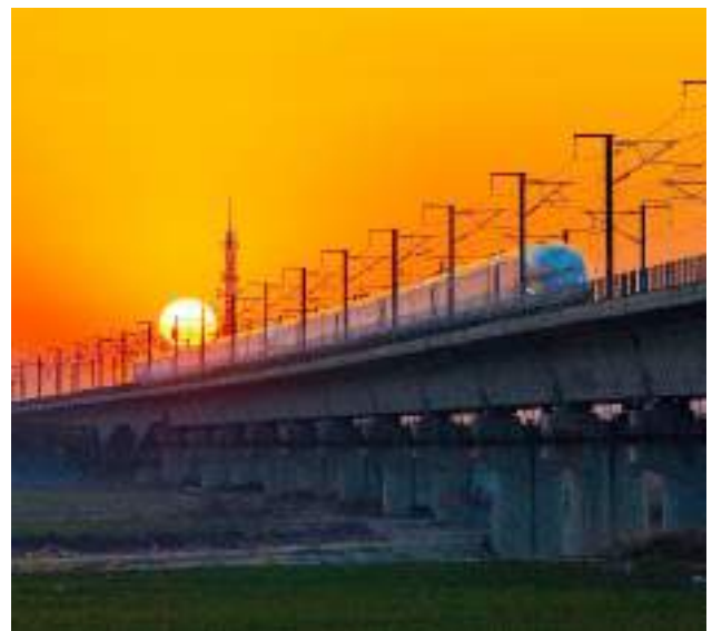
A5 Beijing-Guangzhou HSR: With a total length of 2,281 km and a design speed of 350 km/h, the Beijing-Guangzhou HSR was put into operation in December 2012. It is the world's longest HSR, running through temperate and subtropical zones, different terrains, geological areas and multiple river systems.
