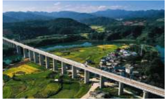
A13 Guiyang-Nanning HSR: With a total length of 482 km and a design speed of 350 km/h, the Guiyang-Nanning HSR opened to traffic in August 2023. 80% of the railway traverses karst areas, connecting more than 30 ethnic minority areas.
