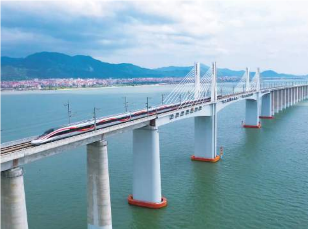
A14 Fuzhou-Xiamen HSR: In September 2023, the 277-km-long Fuzhou-Xiamen HSR, China's first cross-sea HSR with a design speed of 350 km/h, was put into operation.
